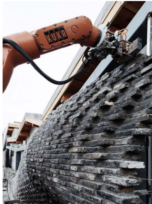
Fig1. Robotic Bricks-laying at ChiShe
